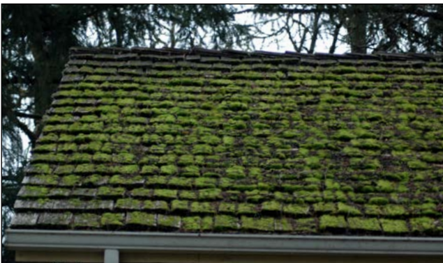
Figure 5a. Moss builds up quickly when roofs are shaded by trees.
