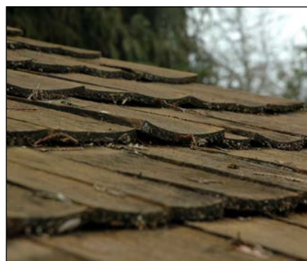
Figure 3b. Cupping and shrinkage of cedar shingles.
