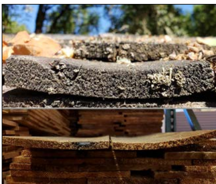
Figure 3a. Cupping of cedar shingles.
