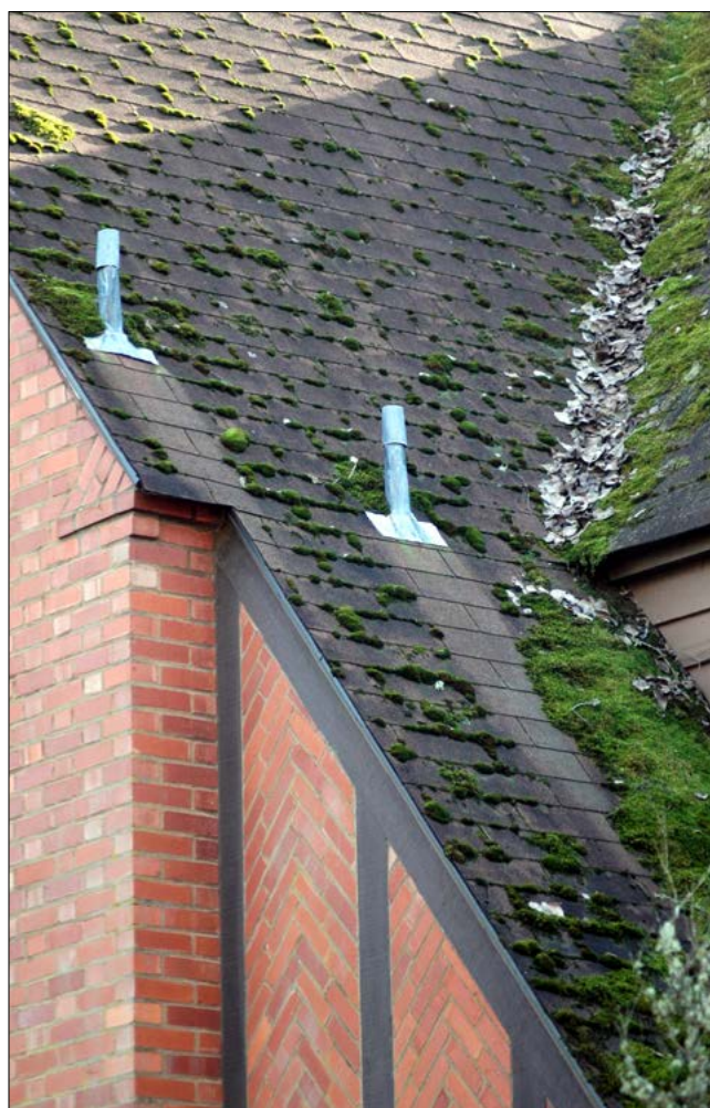
Figure 8. Metal flashings have prevented the growth of moss where water flows beneath the fixtures.
