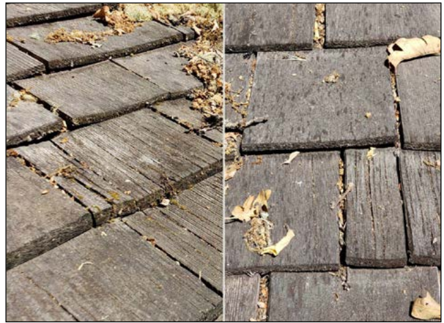
Figure 2. Examples of weathered western redcedar shingles.
