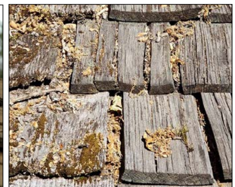
Figure 3c. Splitting and shrinkage of cedar shingles.
