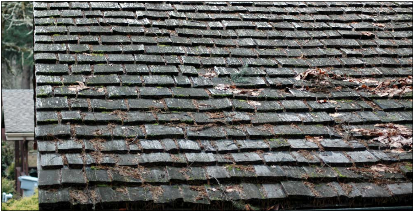
Figure 6. Remove all leaf litter, conifer needles, and debris that accumulate between the shingles and shakes and in the valleys. It's best to do this before the wet season begins.
