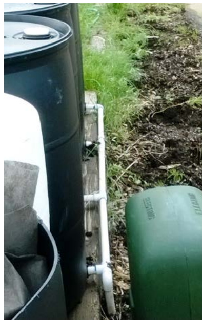
Figure 10a. Common food-grade, 55-gallon barrels can be used for collecting rainwater. Sometimes the primary barrel is linked with others to expand rainwater collection and storage. Barrels should be covered and have vents screened to discourage infestation.
