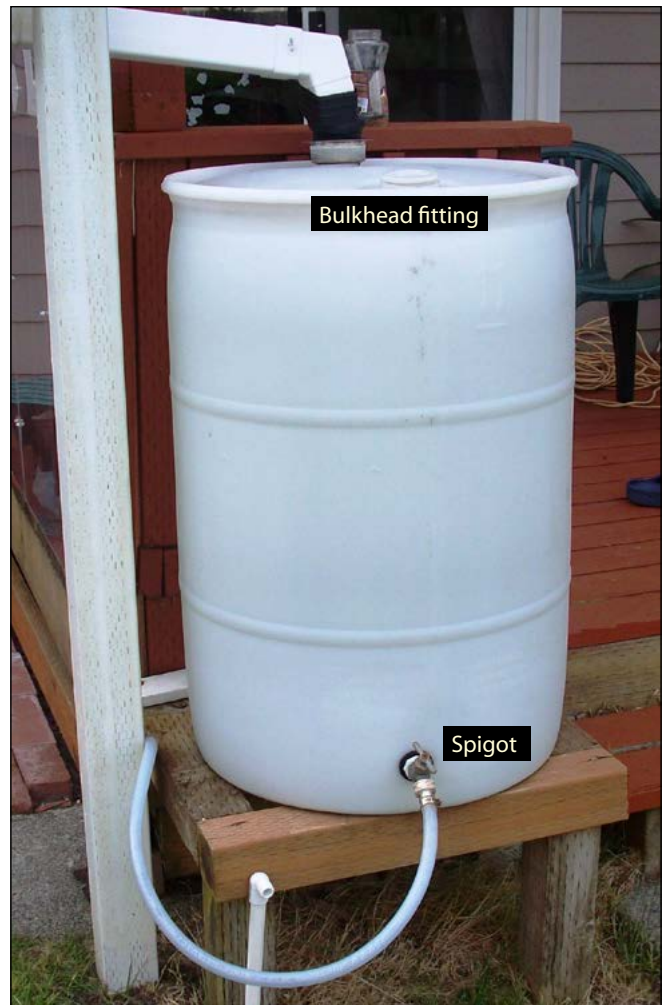
Figure 11. Commercially available rain barrels are fitted with a bulkhead fitting and spigot for garden watering.
