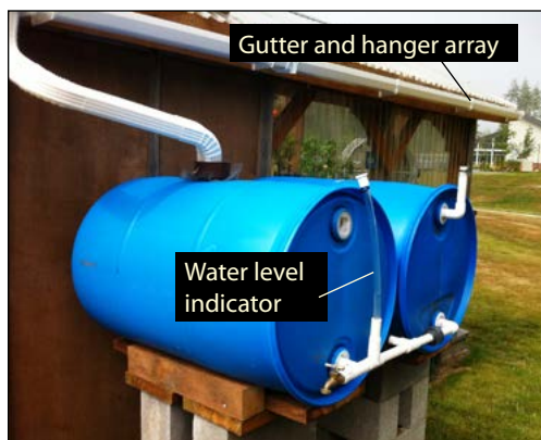
Figure 10d. Gutter and gutter-hanger array for conveying rainwater to storage tanks without using a fine-mesh filter. Also showing alternate way to connect two or more food-grade, 55-gallon barrels in a series for rainwater storage and delivery without the need for a pump.
