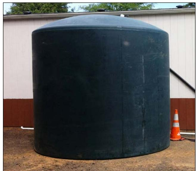
**Figure 12.** Polypropylene water storage tank with a 10,000-gallon capacity.
