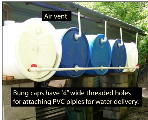
Figure 10c. Alternate way to connect food-grade, 55-gallon barrels in a series for rainwater storage and delivery. Bung caps used for securing contents of the barrels have \frac{3}{4} -inch pipe threads to easily connect PVC pipes for water delivery.
