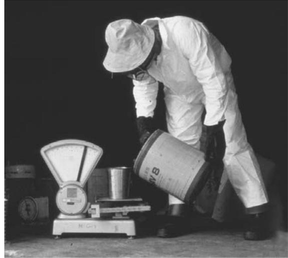
Figure 8. Pesticide handlers must wear appropriate protective clothing, as indicated on the product label.
