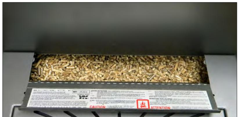
Figure 5. Wood pellets in a pellet stove hopper.
