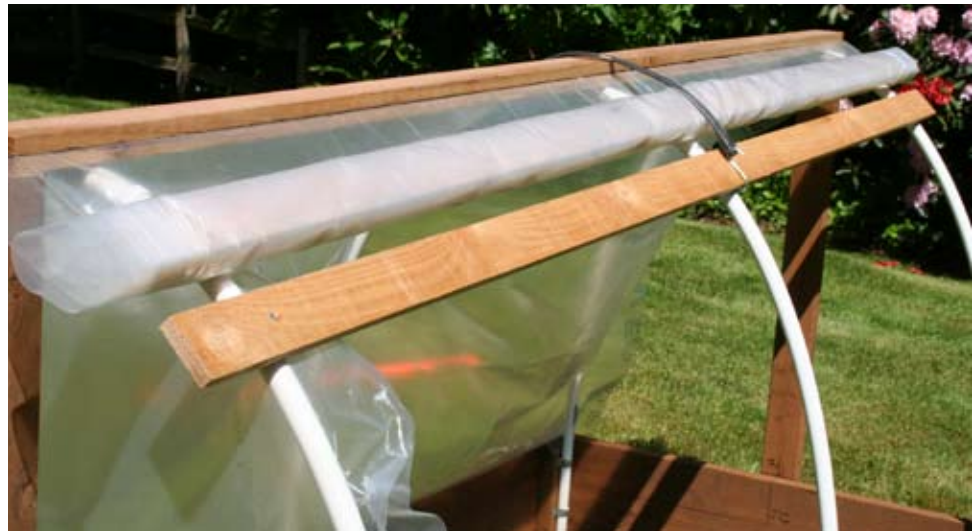
Figure 11. A D board attached to all the hoops 10 inches below the backbone on each side gives the structure extra strength and support.
