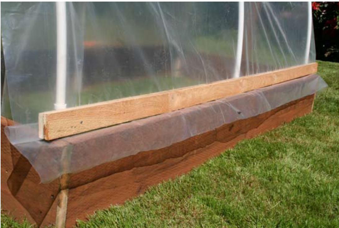
Figure 10. Secure the side curtain plastic with two D boards that sandwich the plastic and rest on top of the raised bed. Trim excess plastic, but leave 6 to 8 inches of overhang.
