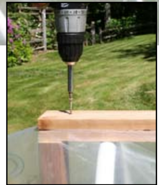
Figure 9 insert. Secure the plastic with 1.5-inch screws.
