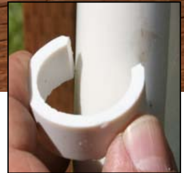
Figure 7 insert. Attach PVC clips to hoop.
