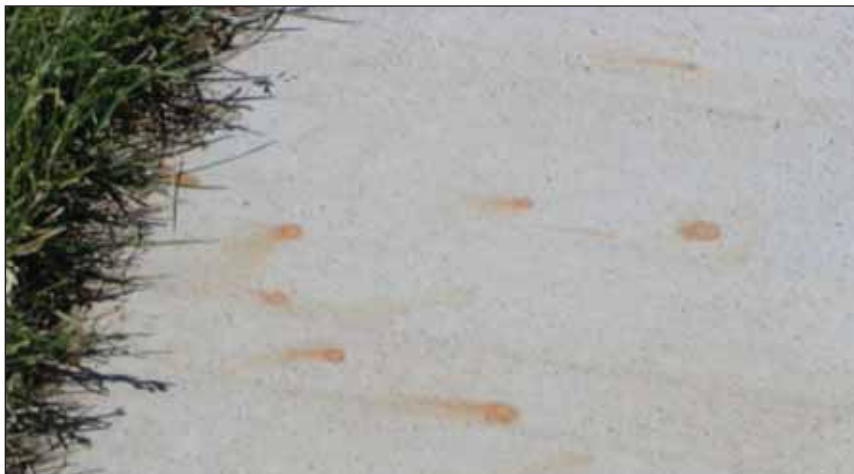
Figure 4. Brown rust stains where iron contacted concrete and then was watered in.
